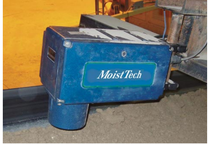
Typical online, dusty installation
